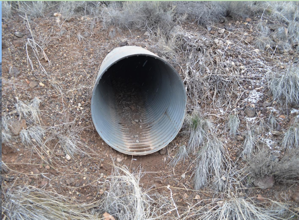
Figure 5: 36" Corrugated Metal Pipe Culvert I
