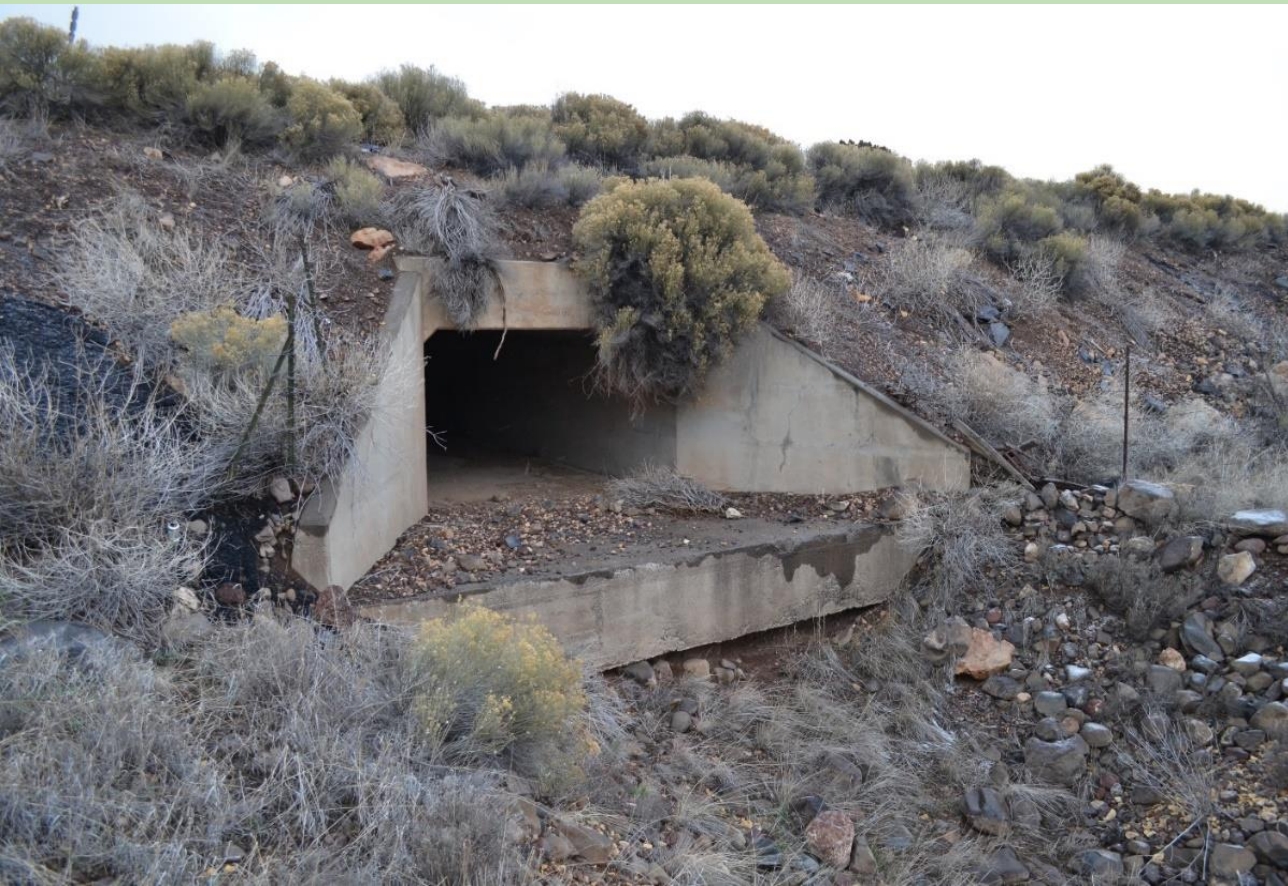
Figure 6: 10'x6' Single Box Concrete Culvert H
