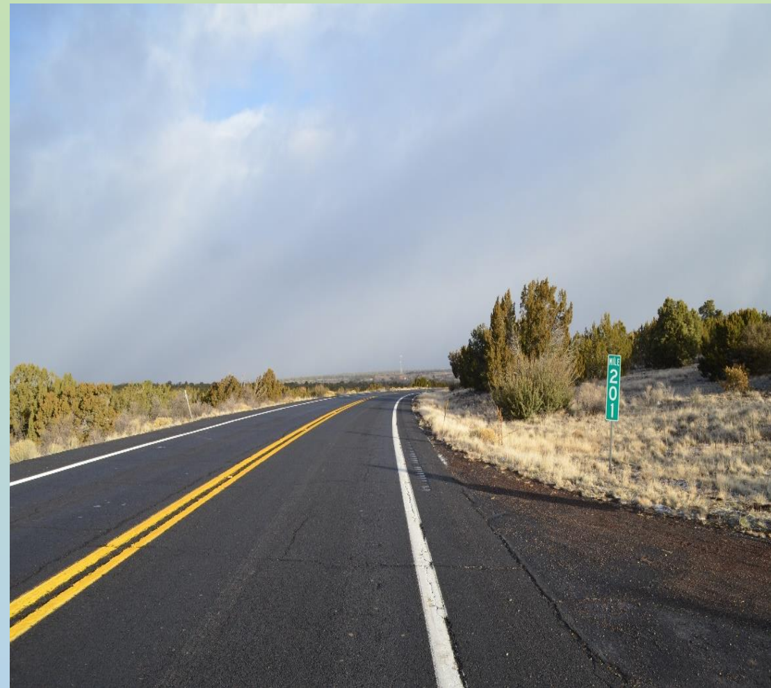
Figure 3: Northbound Mile Marker 201 View
