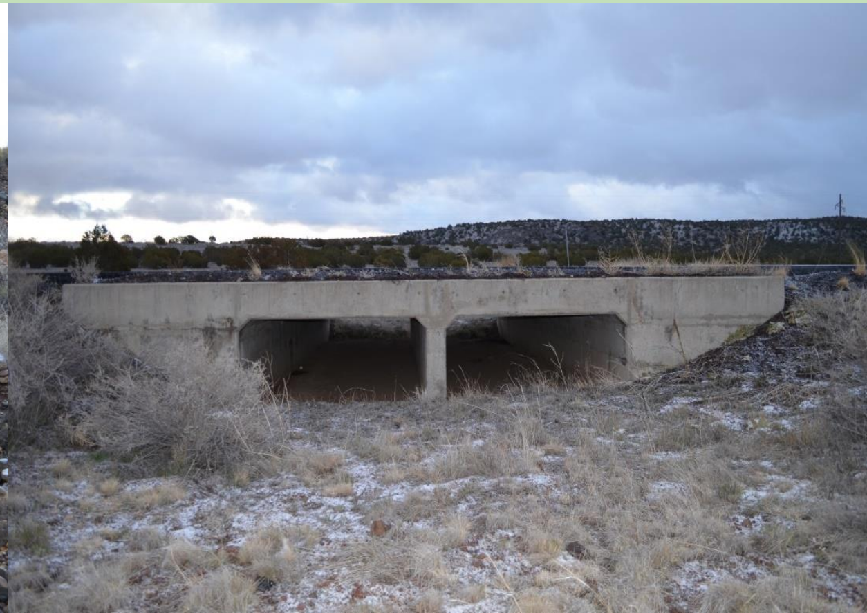
Figure 7: 8'x4' Doubled Box Concrete Culvert F
