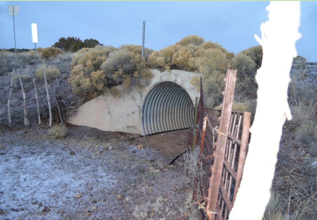
Figure 4: 78" Corrugated Metal Pipe Culvert A
